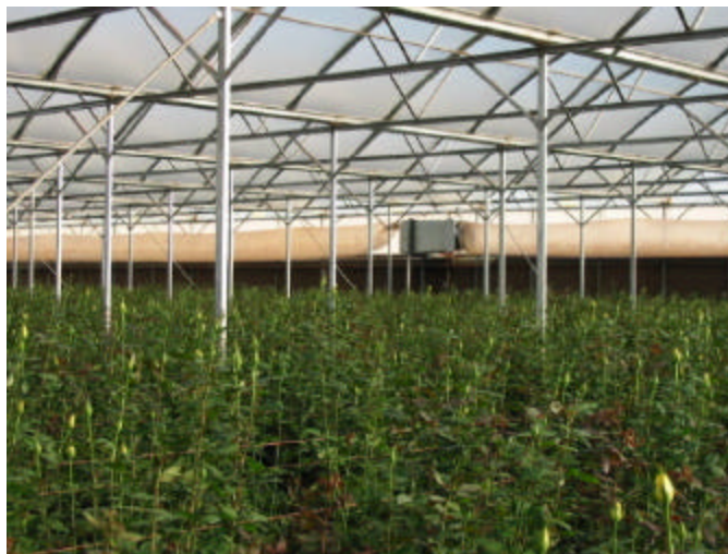
Inside View (visible on the far side is a "wet wall" for cooling and a dehumidifier system)
