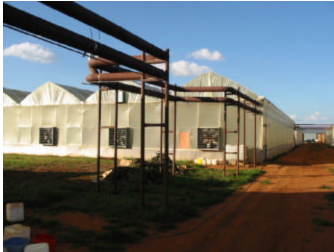
Outside View of the Greenhouses
